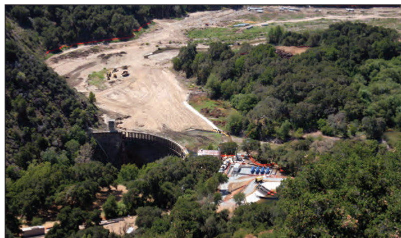
Silt accumulation in the old Carmel River stream bed above San Clemente Dam – Joe McCarthy
