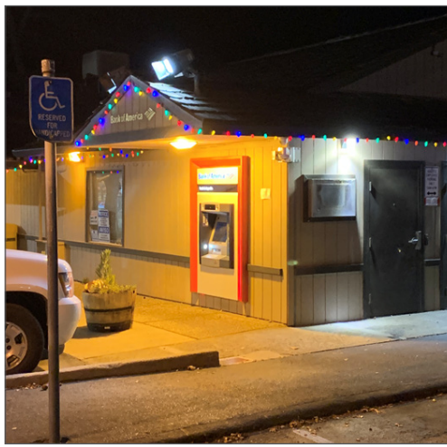
"Barn door" fixtures for lighting over ATM focus light just where it's needed. Photos by John Heyl
