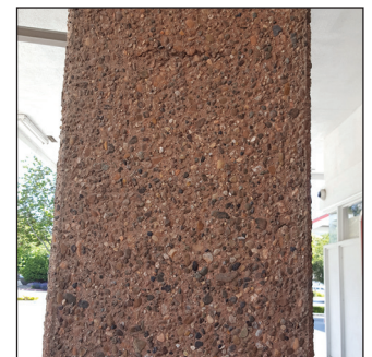
Left, some of the columns painted white prior to permitting, right, an original exposed aggregate column.
