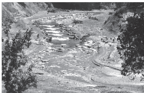
Step pools facilitate steelhead migration upstream from demolished dam — photo by Mibs McCarthy
